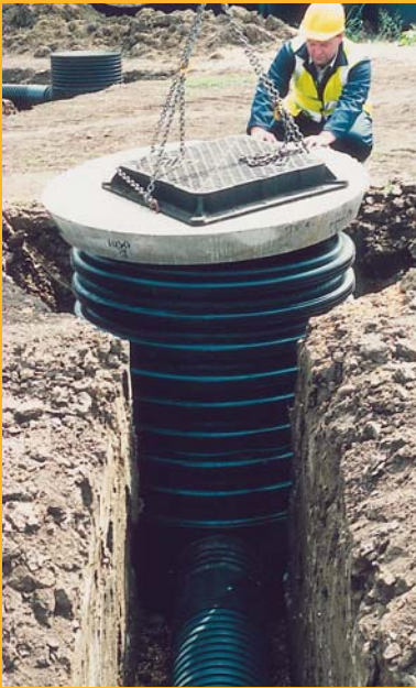
Cover slab and cover placed in the traditional way
