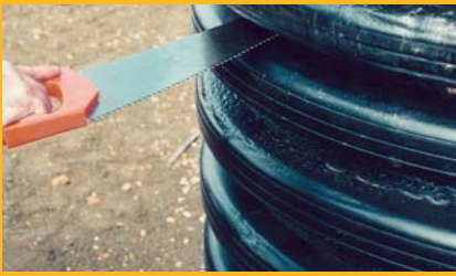
Rising sections or single piece manholes are easily cut to the required length
