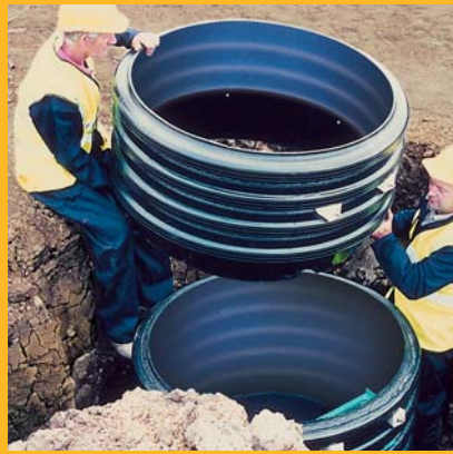
Rising section keys into the manhole base section
