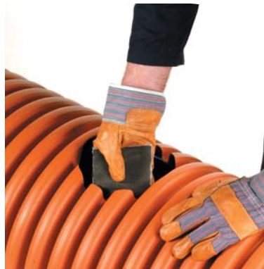
STEP 2 → Sand down the rough edges of the hole
