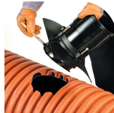
STEP 3 → Apply Polypipe lubricant to the seal
