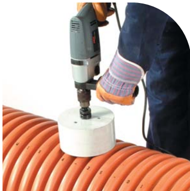
STEP 1 → Cut the hole in the pipe using a suitable drill
