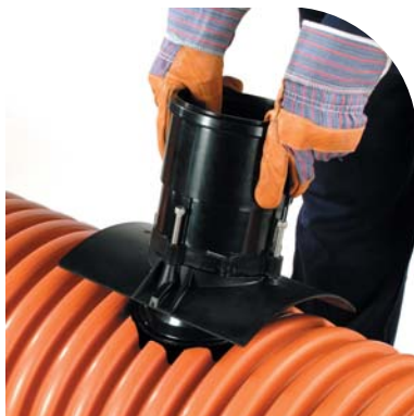
STEP 4 → Push the saddle connector firmly into the hole
